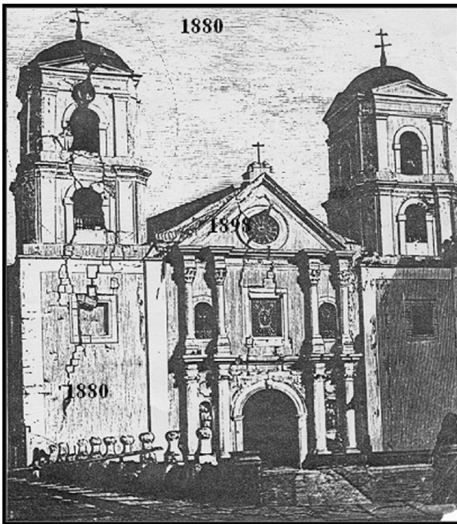
(b) past damage condition
