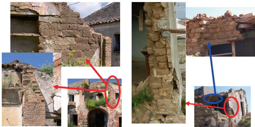
Fig. 4.5.6 Examples of adobe walls
